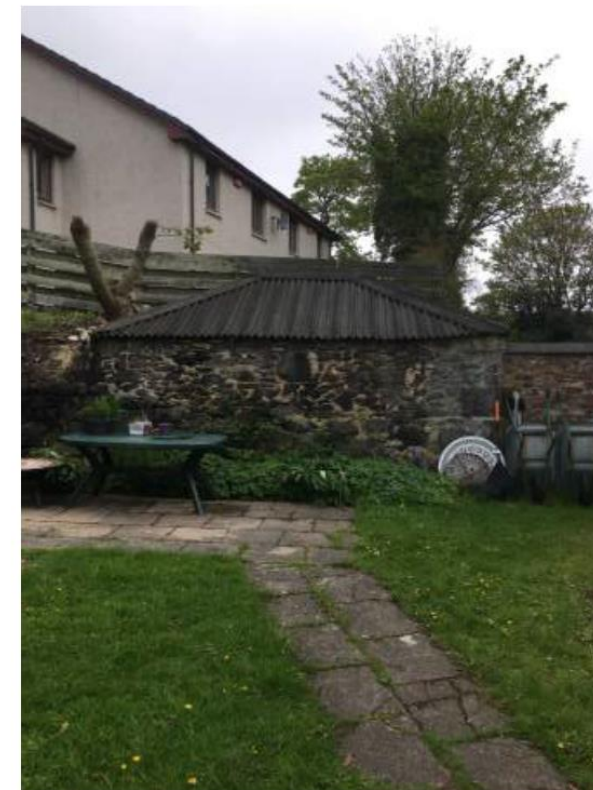
GARAGE WEST WALL
